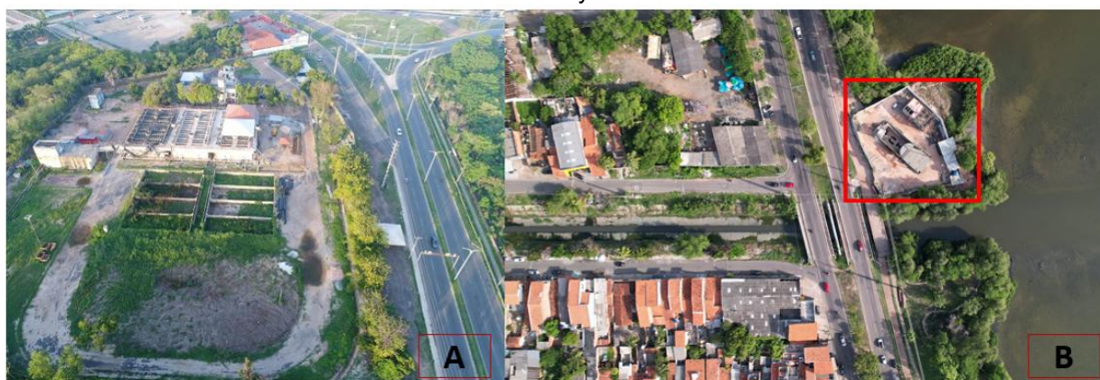
Figure 4. (A) Aerial view of the Bacanga Wastewater Treatment Plant (WWTP); (B) Sewage Pumping Station (SPS) located on Avenida dos Africanos, both components of the Bacanga Basin wastewater system.
